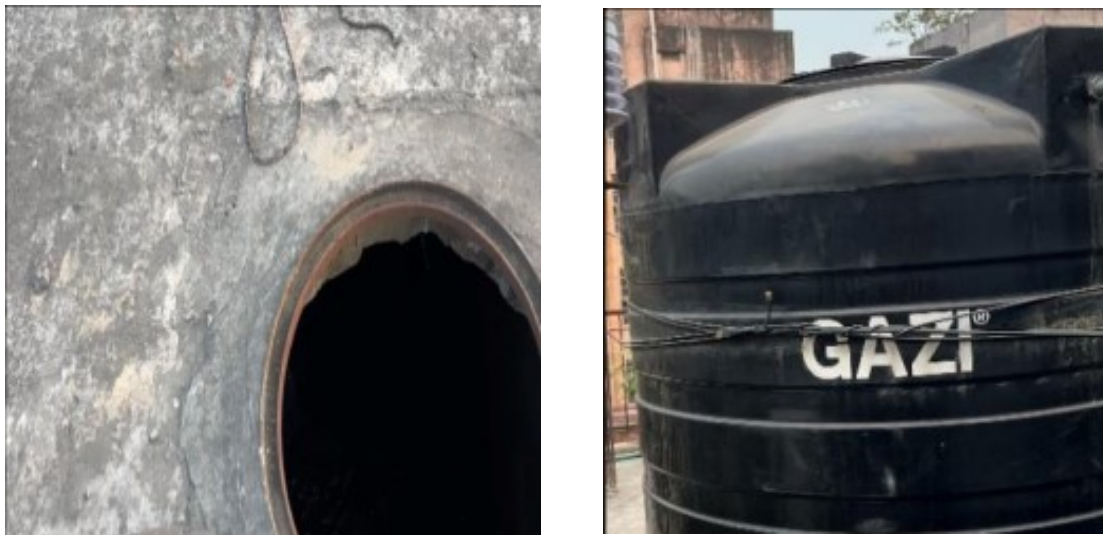
Figure 2: Overhead tanks: (a) RCC tank at Dhanmondi; (b) Plastic tank at Mirpur
