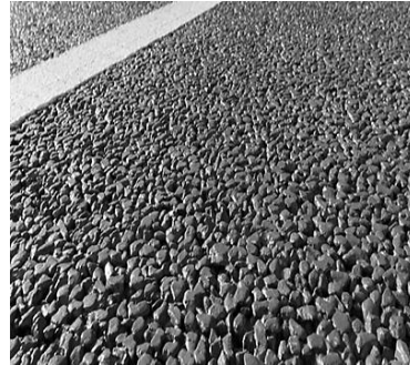
Figure 9: Pervious pavement
