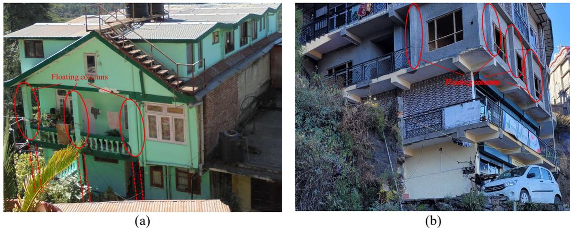
Fig. 1. Hill buildings with floating columns
