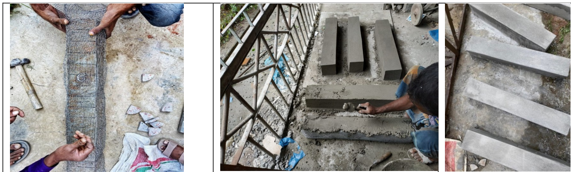
Figure 3.1.3 Columns after ferrocement jacketing with single layer.
