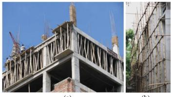
(a) (b) Figure 10: Bamboo poles used for construction (a) propping (Mukul & Rana, 2013) and (b) temporary formworks (Riyad, 2023)
