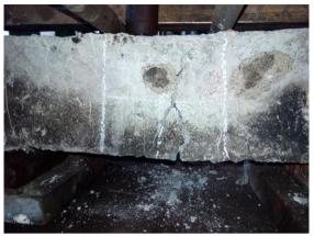
Figure 5: Spalling of concrete in the beam due to burning in fire.
