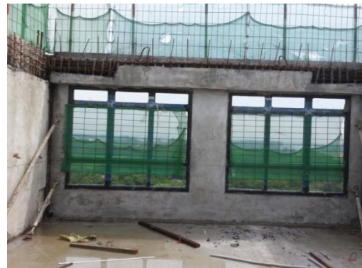
Figure 11: Façade panel being installed
