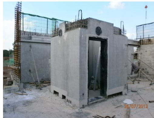
Figure 19: After installation of household shelter
