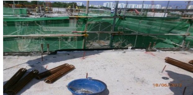
Figure 9: Bedding preparation for façade installation
