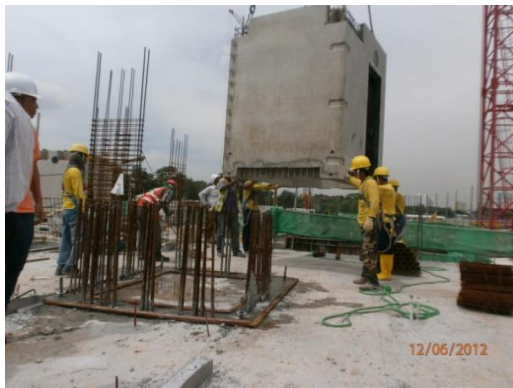
Figure 18: Installation of household shelter in progress
