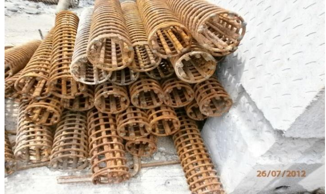
Figure 5: Spiral connector for column or wall connection
