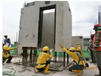
Figure 23: High quality workmanship using PPVC
