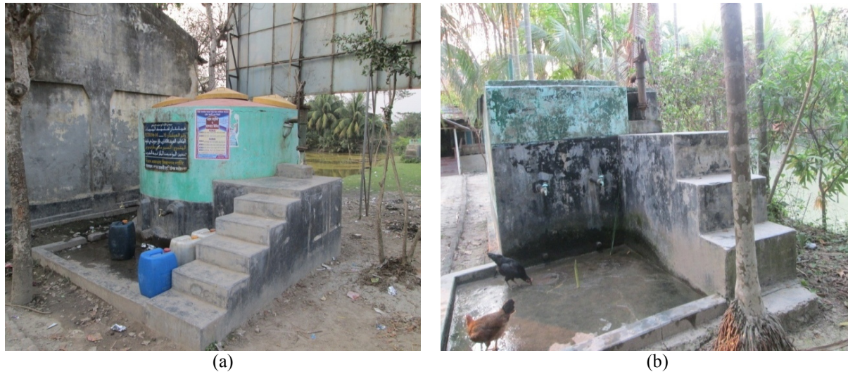
Figure 12: Pond Sand Filter in (a) Morrelganj (April, 2013) and (b) Kaliganj (August, 2013)
