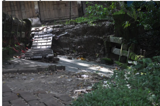
b) Broken culvert
