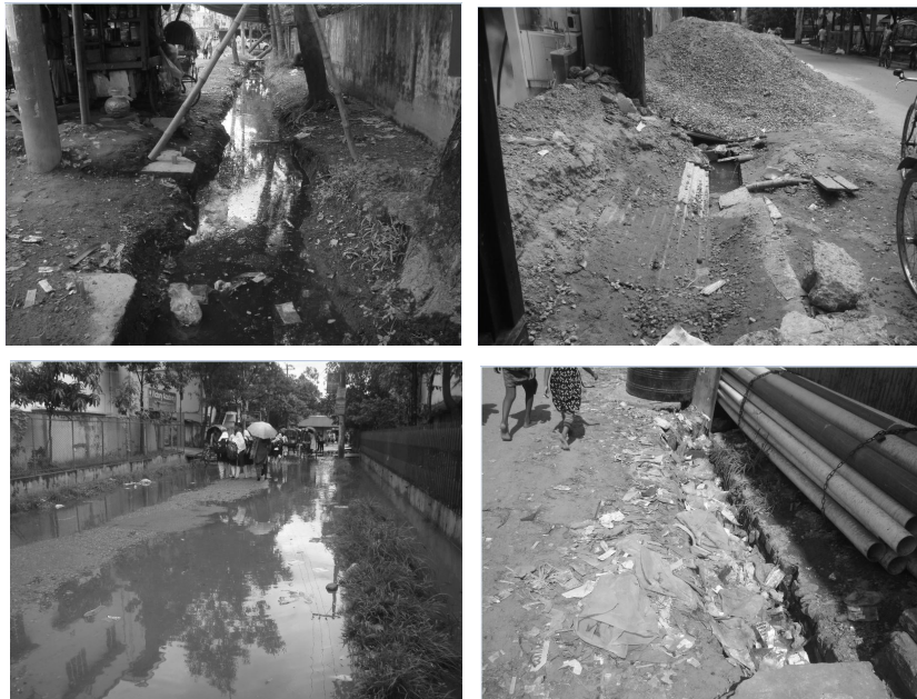
Figure 6: Condition of tertiary drains
