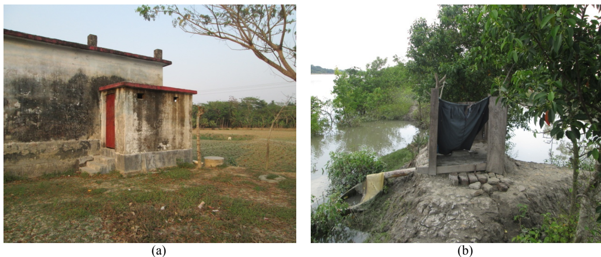
Figure 13: Existing sanitation system (a) community sanitary toilet in Morrelganj (April, 2013) and (b) hanging toilet in Kaliganj (August, 2013)
