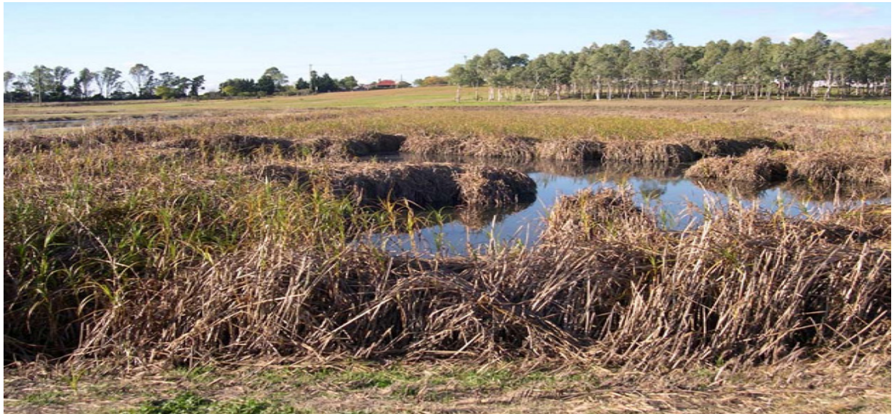
Figure 2.3.1: A FWS CW for tertiary treatment of municipal wastewater in McGrath Hill, Hawkesbury, near Sydney, NSW, Australia.
