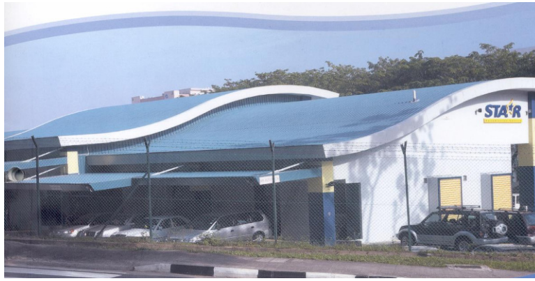
Figure 2: Profiled steel sheet roofing element in Singapore (Bluescope- Lysaght, 2003)
