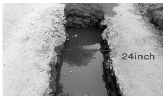
Figure 2: A photograph of a trench for laying pipe line
