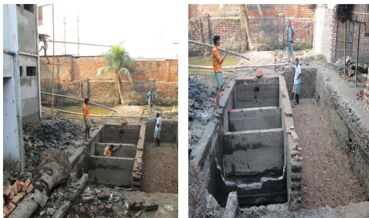
Figure 2: Construction of Decentralized Wastewater Treatment Plant of D4 Building
